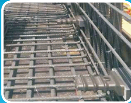
FIXING OF BURSTING LINKS
