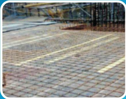
LAYING & PROFILING OF TENDONS
