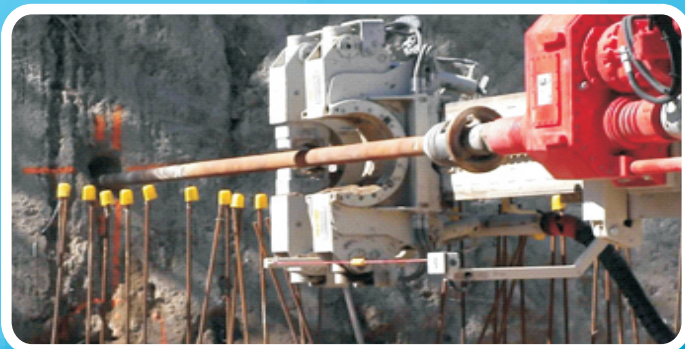
FABRICATION OF ANCHORS
