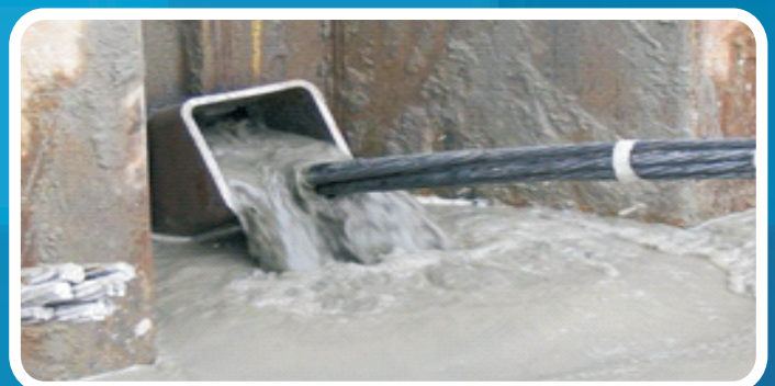
GROUTING OF ANCHORS
