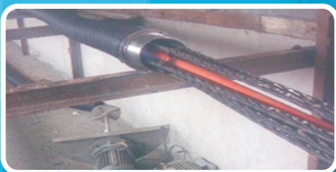
FABRICATION OF ANCHORS
